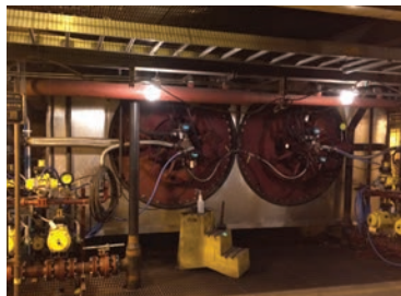
Two of four low NOx burners installed on Orrville's largest 25 MW generating unit.
